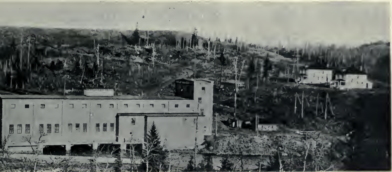
ks, Reinforced Concrete Power House and Tall Race—Kamlnistqla River in Foreground and Transmisston Ltne to the Right.
